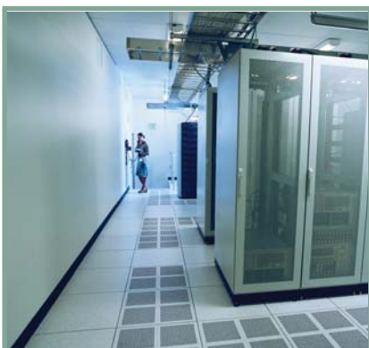
Precision Air Conditioning
